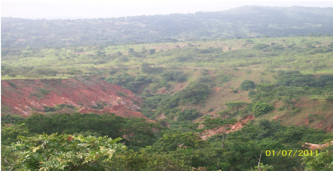
Fig 2 Gully site at Ukana, Enugu State
